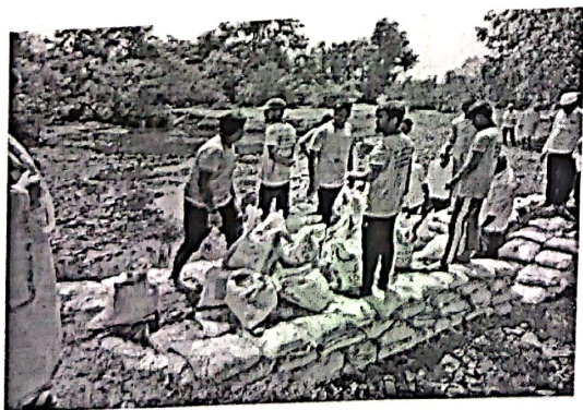
Two Bandhara (Temporary Soil Sack Dam) on River (Takeshwar - Dhasai Forest Dept.)
